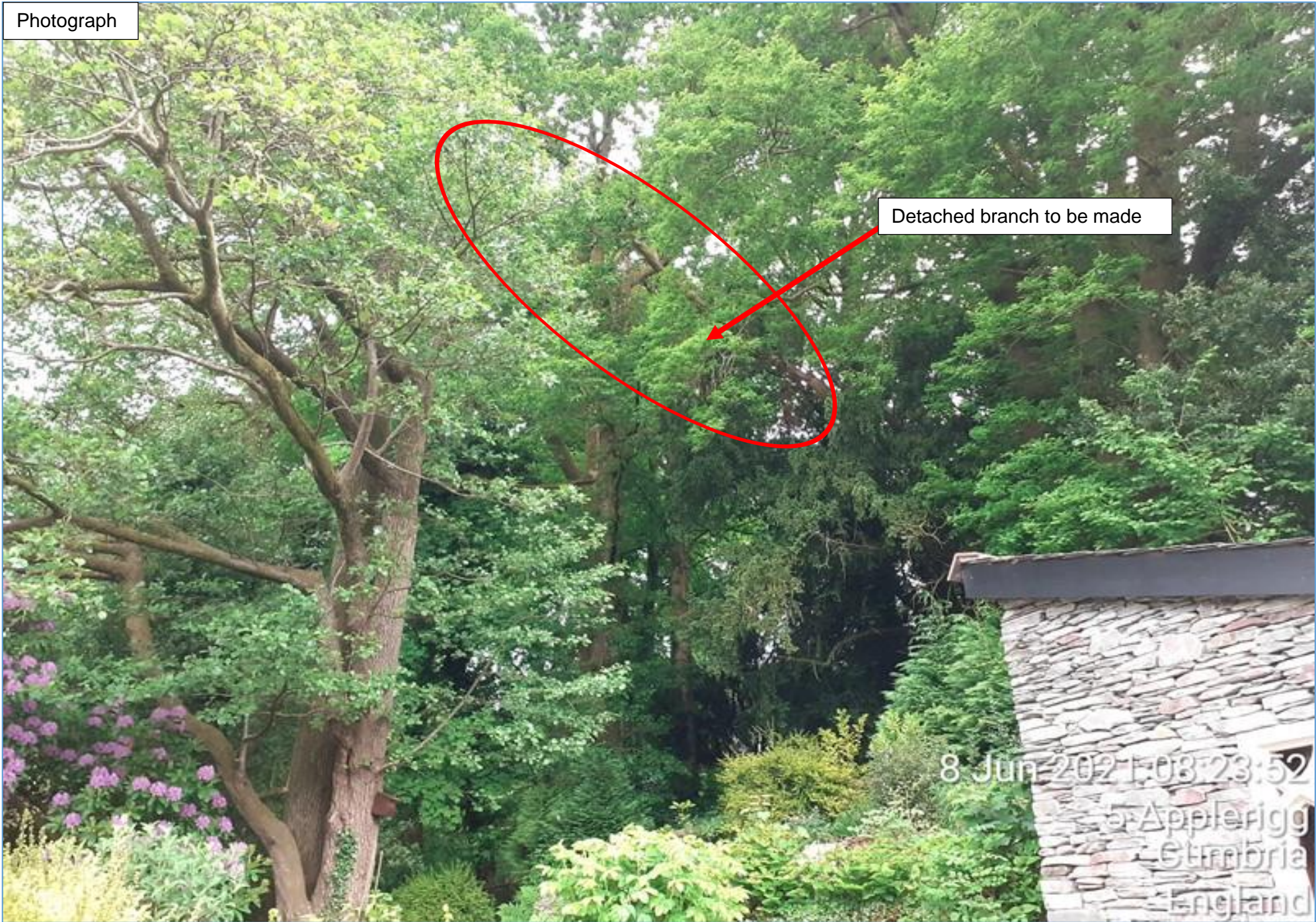
Photograph 1 showing the detached branch to be made safe - viewed from The Lodge, Wynlass Beck.
